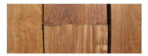
For butt joints, whether face or blind fastened, it's essential to block by adding a sister joist or double 2x stringers. This approach ensures proper fastener placement and prevents positioning fasteners too close to a butt joint, which can happen when trying to attach both boards to a single joist.
