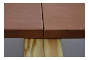
Additionally, some contractors use biscuits or dowels to eliminate any potential movement at the butt joints. Utilize hidden fasteners that create a mechanical connection between both pieces of decking and the stringers to maintain even spacing and prevent the boards from moving, as illustrated below.
